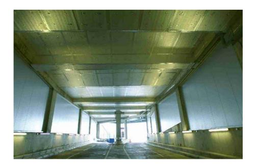
Kingspan Kooltherm K10 Soffit Board was installed to thermally insulate between the B1 car park level and the ground floor of the new building known as 5 Churchill Place part of the prestigious Canary Wharf development, London.
